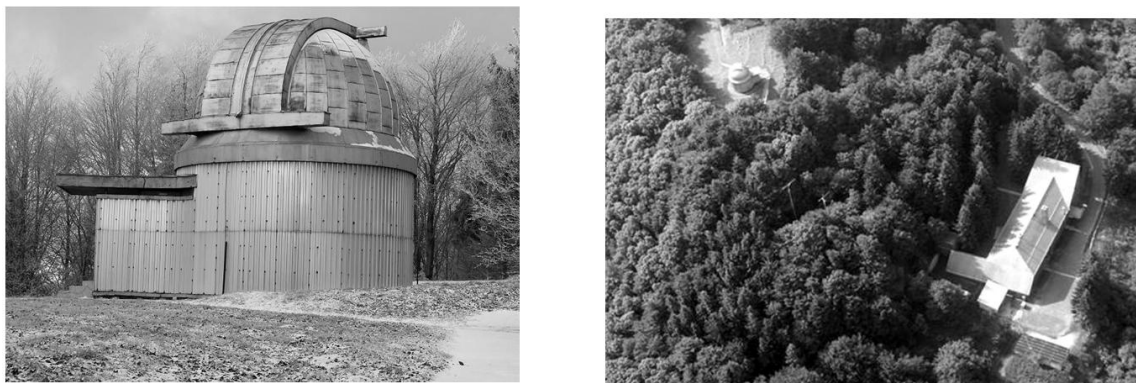
Figure 8: The dome of the 50 cm telescope and its aerial view (with the main building)
